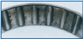
TOO LOOSE, RESULTING IN VIBRATION OR FALSE BRINELLING (SHOWN) OF THE BEARING OR RACES
